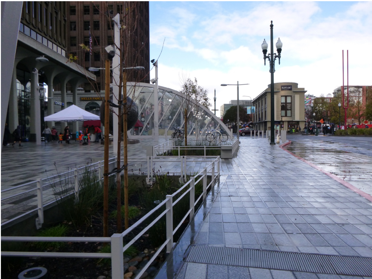
Figure 33 – Flow-through planters installed above the Downtown Berkeley BART Station treat runoff from Shattuck Avenue.
