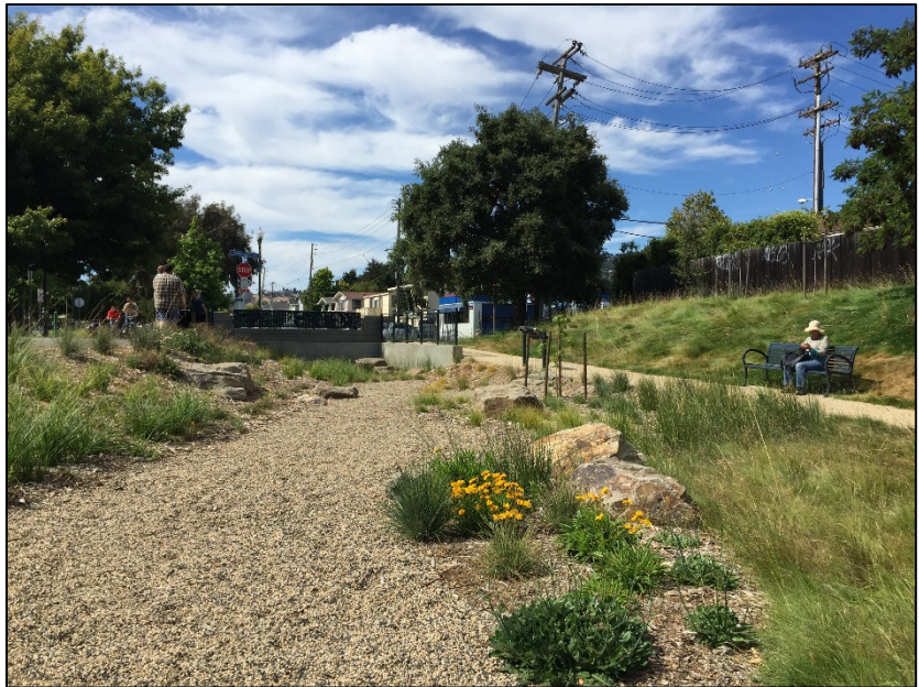
Figure C-6. Ohlone Greenway Natural Area and Rain Garden. This rain garden captures and treats runoff from an adjacent segment of Fairmont Boulevard. In this instance, the rain garden location provided an opportunity to convey and treat stormwater outside the street right-of-way. Source: PlaceWorks
