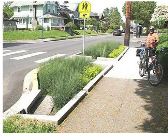
Figure 3-8, Vegetated Swale at Curb Extension
