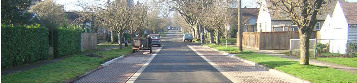
Figure 3-8, Pervious Joint Paving in Parking Lanes of Residential Street
